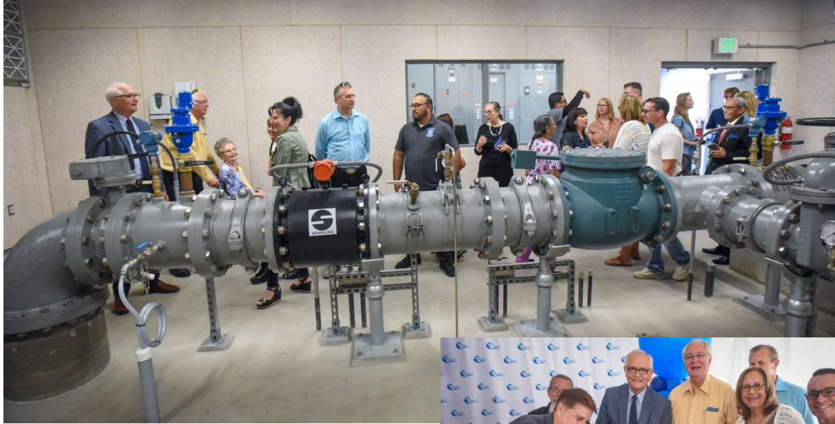
Leahy Well Dedication attendees tour the pump house.
